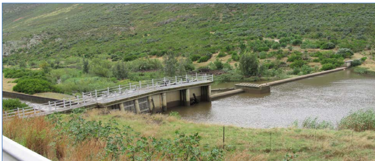
Figure 3: The Existing Klein Berg Diversion Weir
